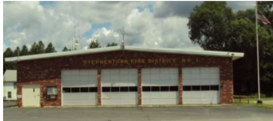
Photo 17: Stephentown Fire District Fire House on NY 43.
