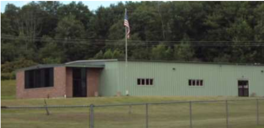
Photo 18: Stephentown Volunteer Fire Department Fire Hall on Grange Hall Road.
