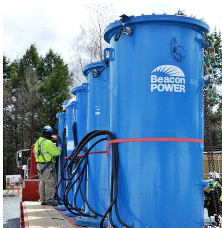
Photo 5: Several of Beacon Power's flywheel power storage units prior to installation.
