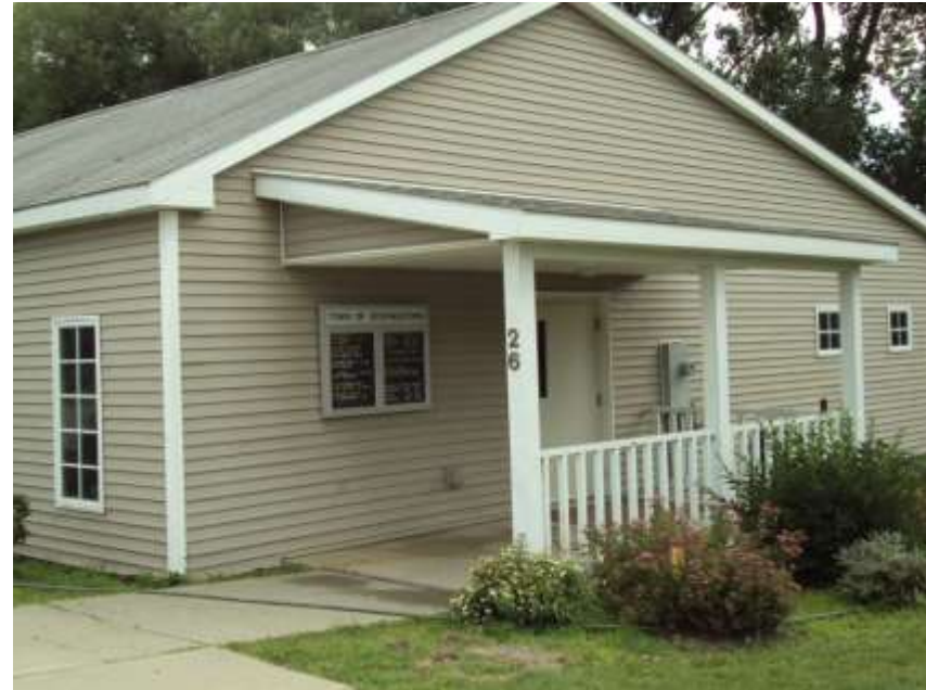
Photo 19: Stephentown Town Hall on Grange Hall Road.
